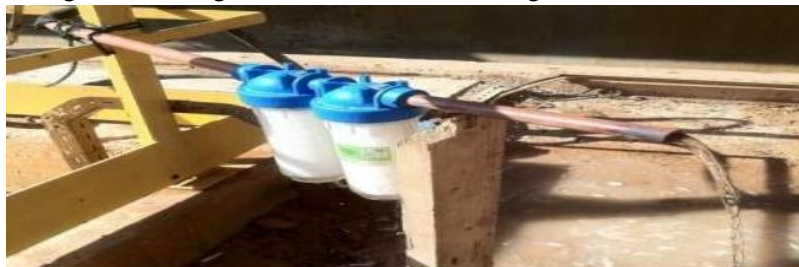
Figure (1) Micro-Filtration setup connected to cooling system blowdown.
